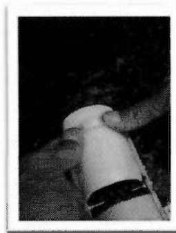
Figure 82: Mould the cable blocks 4
